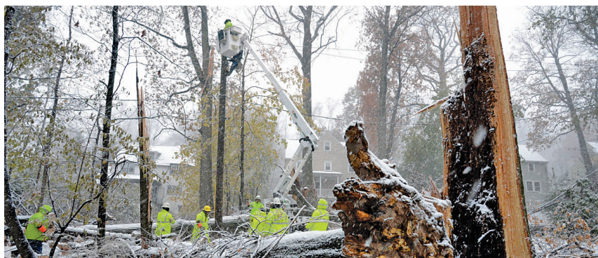
FPL workers help restore power in the aftermath of Hurricane Sandy.
