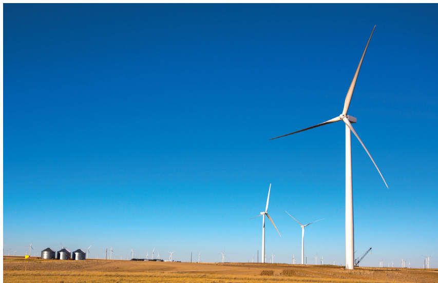
NextEra Energy Resources added more megawatts of U.S. wind in 2012 than any company ever has in a single year, including the Limon II wind facility in Colorado.
